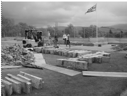
Photo shows the carefully removed stonework prior to refitting..
