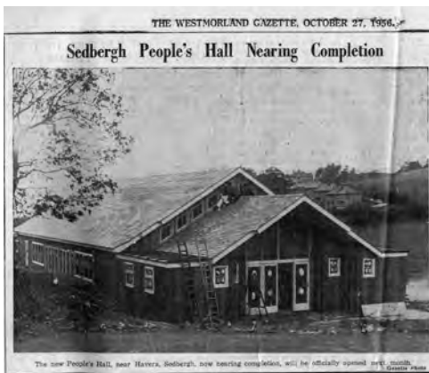
People's Hall under construction in 1956
