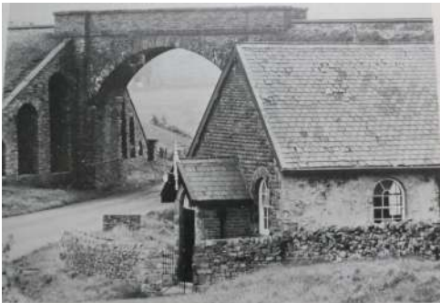
JUNCTION CHAPEL, GARSDALE HEAD, NEXT TO THE RAILWAY VIADUCT. Each hamlet in the Dale came to have its own chapel in the 19th century
